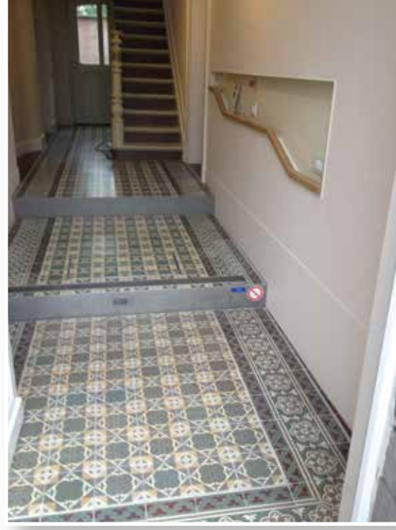
Entrance Hall. Integrated Lift Platform
