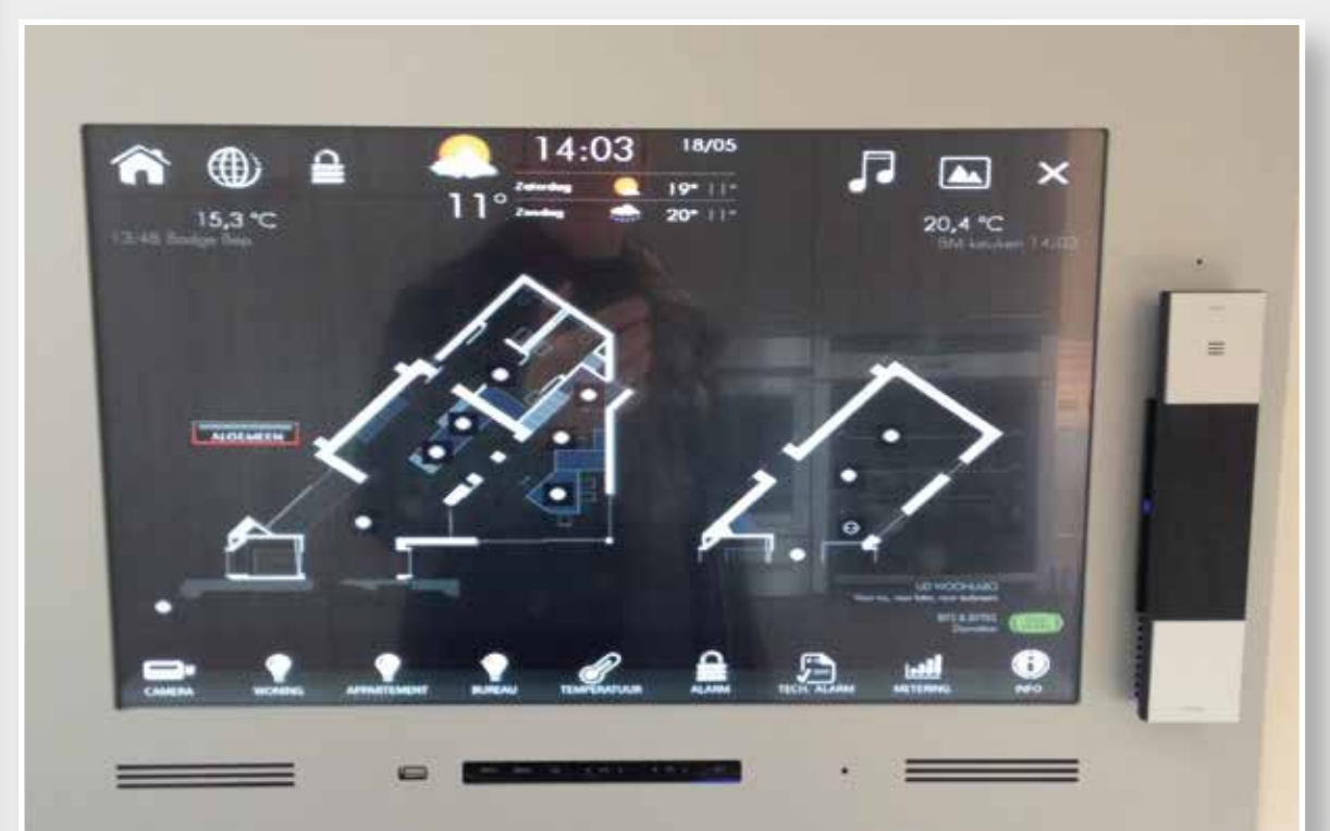
Home Automation System
